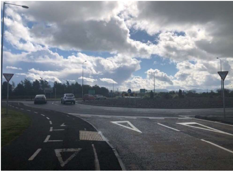
Location 31 - N21 R577 N23 Roundabout
