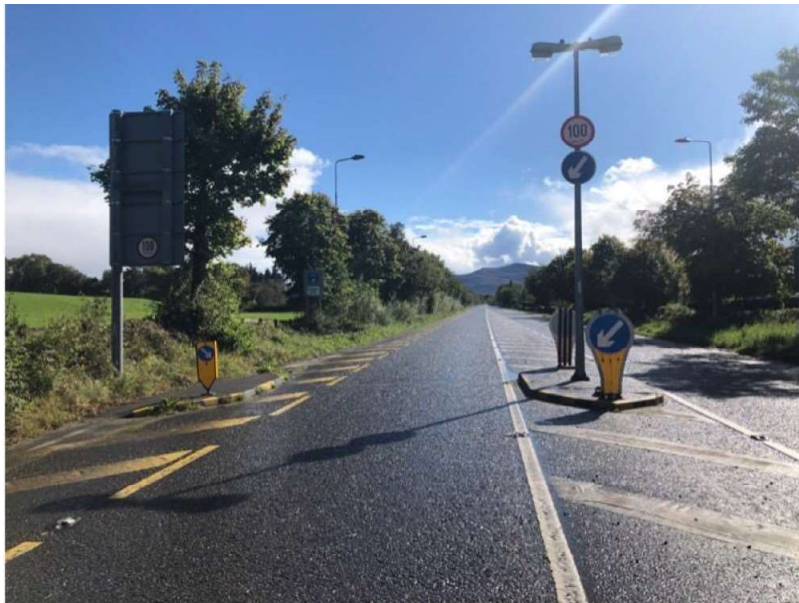
Location 42 - Lissivigeen Splitter Island Exit
