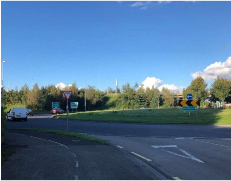
Location 7 - N69/N18 Roundabout Direction Turn Left Onto N18
